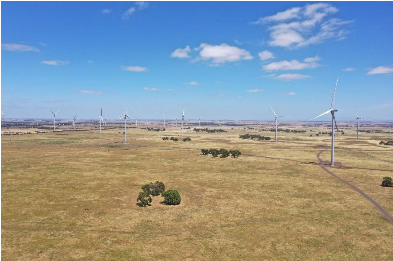
PLATE 1-3 PHOTO OF INSTALLED TURBINES ON SITE, WEST GROUP WEST OF STOCKYARD HILL ROAD, PASTORAL AREA
