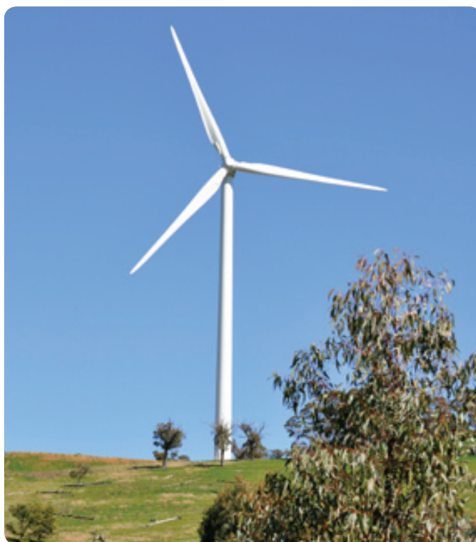
Origin's Cullerin Range Wind Farm, New South Wales.
