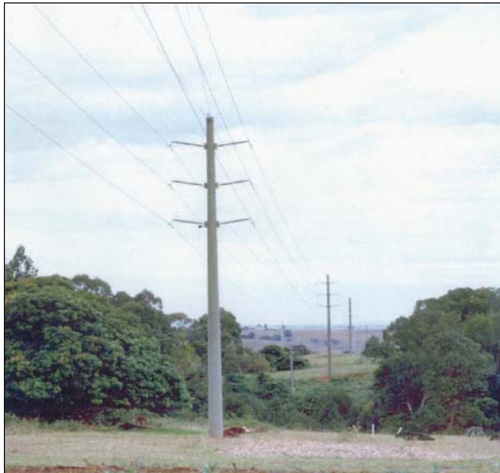
Figure 4.3 Typical double circuit 132kV suspension structure
